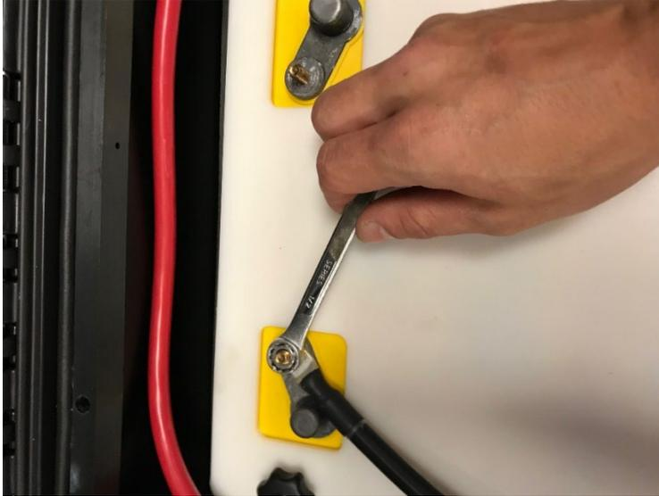
17. Carefully attach the red positive DC cable to the battery that is closest to you. Assure that the terminal shows a (+) symbol. Use a 1/2" wrench to tighten. **Be very careful not to touch the other battery terminals with your wrench.**
